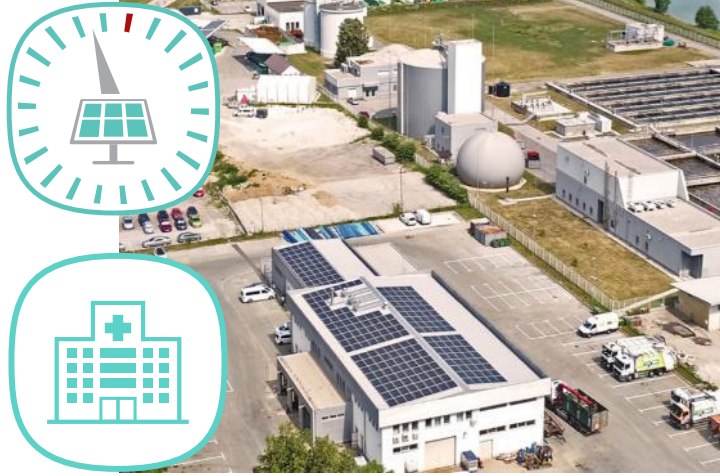
SOLAR POWER PLANTS
